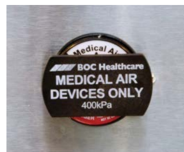
Figure 5: Medical air flowmeters are fitted with a labelled, movable 'guard' that covers the tubing connection to raise awareness of gas selected (left) and air blanking plugs are fitted to all outlets not in use
